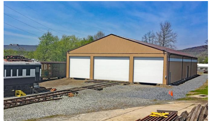
The new rail car protection building at the Reading Railroad Heritage Museum
