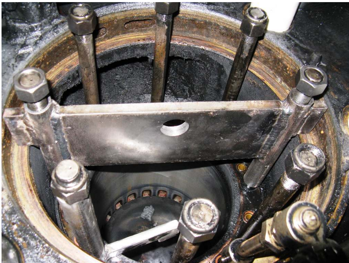
(TOP) With the head removed, we also removed the liner anchor tool. Then the liner jacking tool is used to jack the liner free of its gasket seats.
